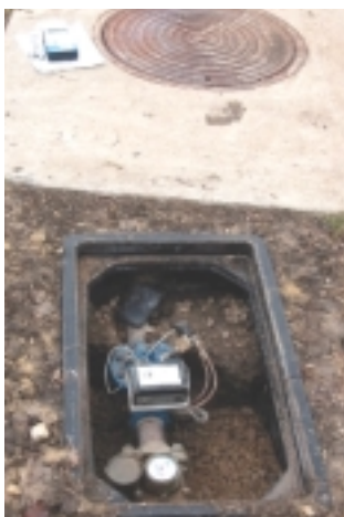
Flushing Valve Installation
