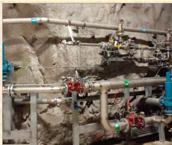
Deep Underground Pressure Reducing Station
