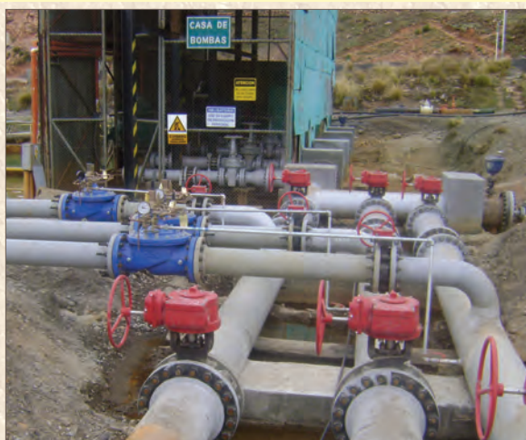
Surge Anticipator/ Pressure Relief Valves and Air Release Valves at Pump Station
