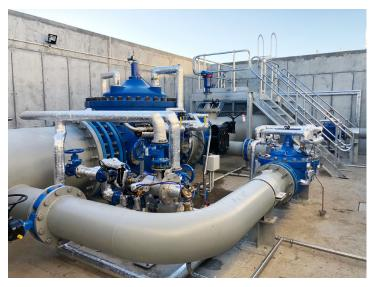
A VC-22D electronic valve controller, controls the operation of the 900mm and 350mm dual solenoid control valves by sending electrical pulses to the opening solenoid, allowing water to flow out from the valve cover chamber, which in turn, allows the valve to open slightly with each pulse, or to the closing solenoid, allowing water to flow into the valve cover chamber, which in turn, allows the valve to close slightly with each pulse. The VC-22D uses a customized ValvApp for the logic controls.
