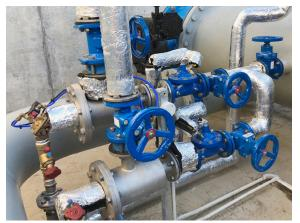
Each PRV stations has three operating states, AUTOMATIC, HYDRAULIC and STATION OFF, which the operator can either set locally or remotely, via SCADA, to operate the PRVs.
