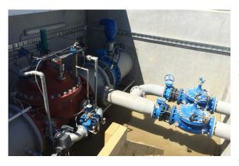
Since the initial piping scheme, the decision has been reached to install a further 124 miles (200 Km) of pipeline, serving an additional 167 properties at a cost of \$95 Million NZD, (\$60.7 M. USD). This also includes Cla-Val control valves for each property ranging is sizes of 1.5" (40 mm) to 14" (350 mm) plus main line electronic control valves in sizes 14", 24", 36" and 40" (350mm, 600mm, 900mm and 1,000mm) along with bypass and relief valves.
