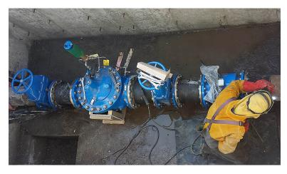
Ten existing 25 year old Cla-Val 90 series valves were fitted with the latest generation of Cla-Vals 34 series actuated pilot controls and 117 series of position transmitters to enable these long serving valves to be upgraded to the latest technology
