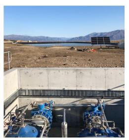
Two 24" (DN600) electronically controlled dual solenoid operated valves with anti-cavitation trim, operating in parallel, will maintain a constant pond level by regulating the filling rate, accordingly, based on the pond's current level and at the same time lowering the pressure to 177 psi (12.2 Bar).
