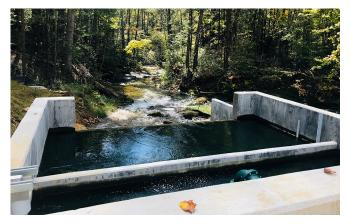
Greenville Water replaced the existing outfall structure with a new weir (left) and added a flow control valve with a customized app (center and right) to automatically control water flow.
