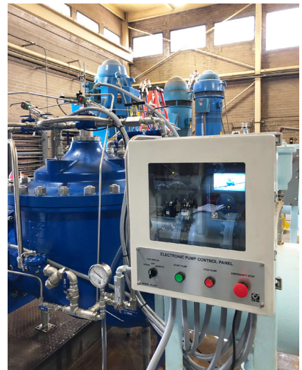
New pump control valve with control panel. Courtesy of Cla-Val.
