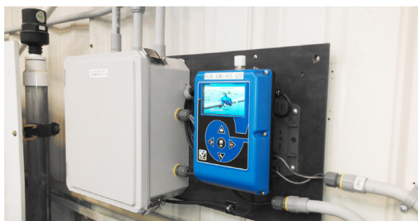
Typical installation with mounting bracket
